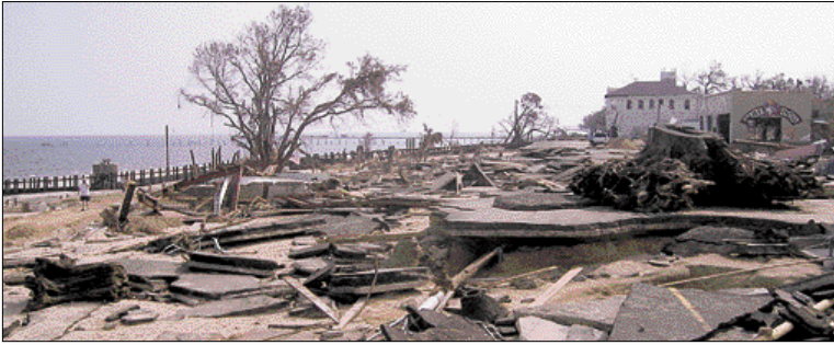
When Hurricane Katrina roared ashore in the Gulf Coast region Aug. 29 as what an Associated Press story termed a "monstrous, 145-mph storm," it brought a storm surge estimated to be more than 30 feet high that destroyed most everything that was in its path. One of the hard-hit areas was Bay St. Louis, Miss., where, according to Tom Garber of Montoursville, state director for Tech Serve International, bridges were knocked off their foundations, roads were crumbled — as evidenced in the photo at left — and up to 60 percent of the homes were destroyed.
